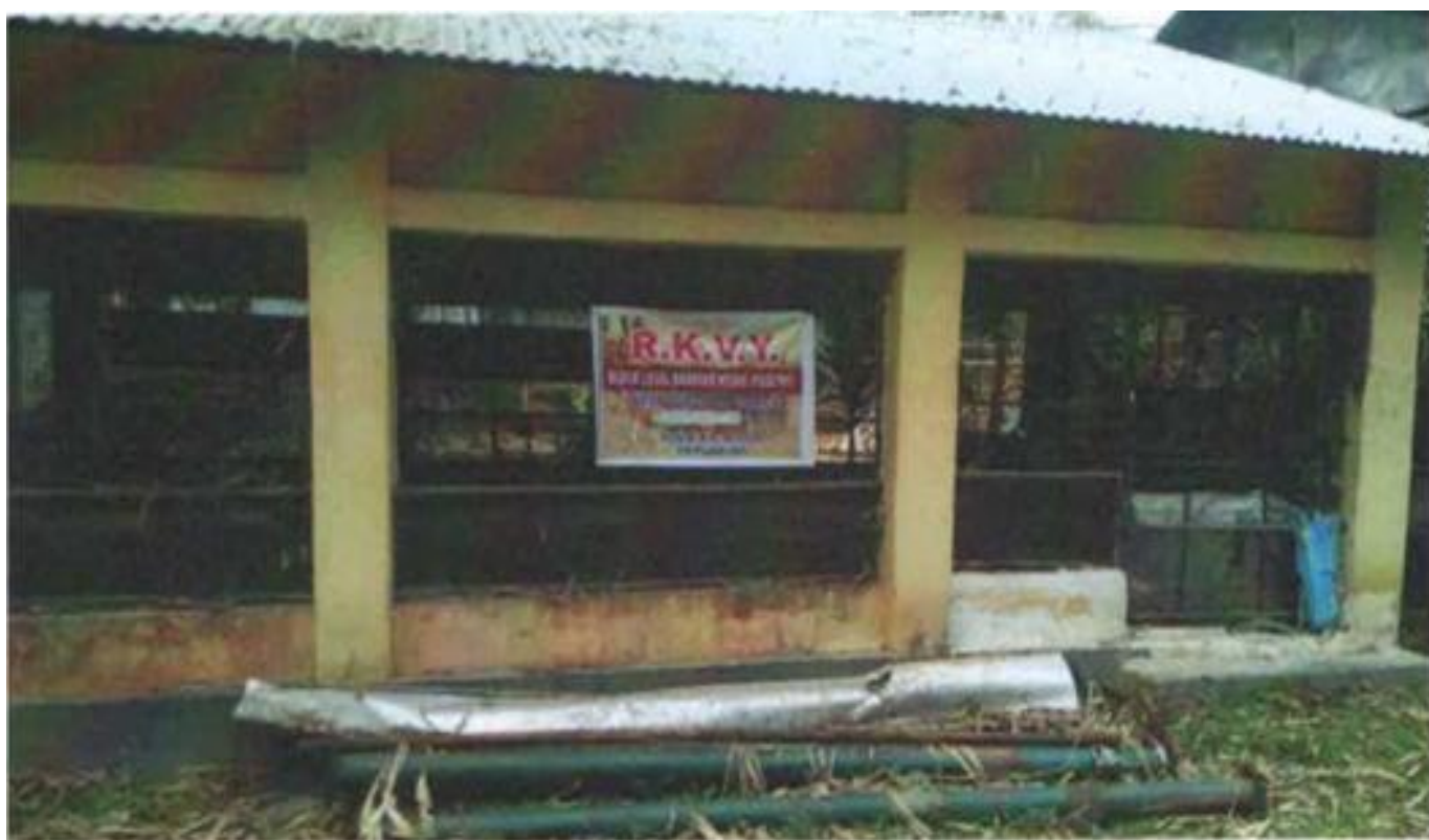
Strengthening of existing brooder House at Durgapur (Dukli R.D. Block) - 2010-11
